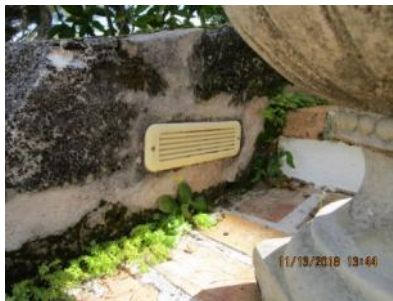
4.91 Recessed louvered fixtures (N) appeared generally sound.
