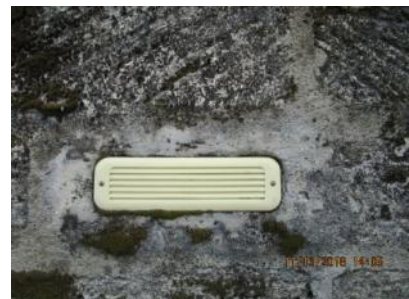
4.101 Recessed louvered fixtures (S) appeared generally sound.
