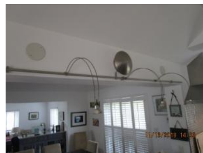
4.35 Wall fixture appeared generally sound.
