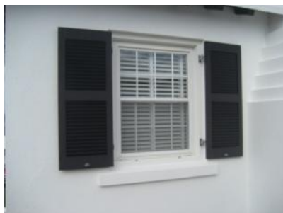
Windows were generally in satisfactory condition.
