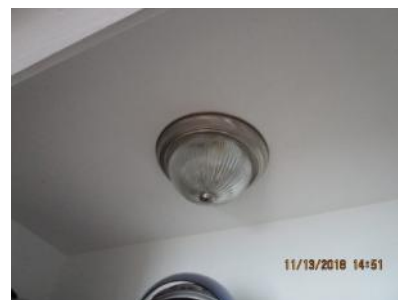
4.83 Closet fixture appeared generally sound.
