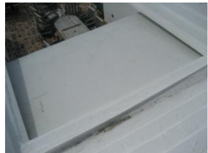
Minor debris accumulation in the valley between roofs.
