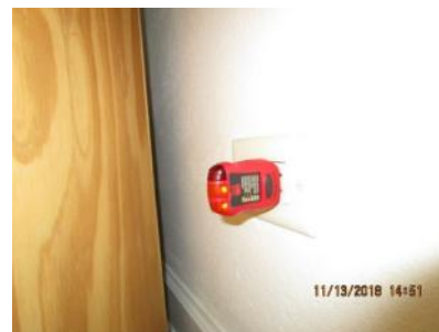
4.80 Receptacle outlet (W) appeared generally sound.
