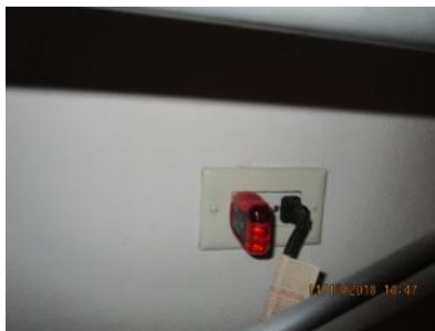
4.70 Receptacle outlet (E) appeared generally sound.
