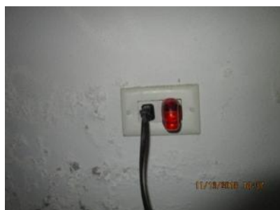
4.45 Receptacle outlet (W) appeared generally sound.
