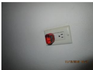
4.15 Receptacle outlet south (W) appeared generally sound.
