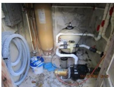
7.17 Pool filter pump appeared generally sound.
