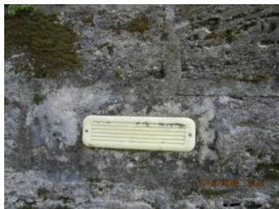
4.99 Recessed louvered fixtures (S) appeared generally sound.
