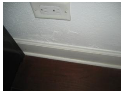
Efflorescence was visible on the east wall.
