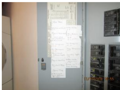
2.3 Panel directory was complete; appeared accurate.
