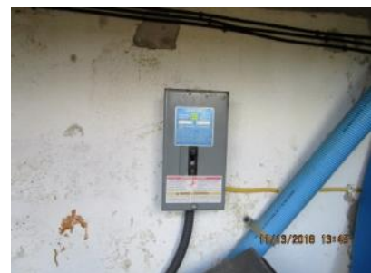
5.4 Disconnect/ circuit breaker appeared generally sound.
