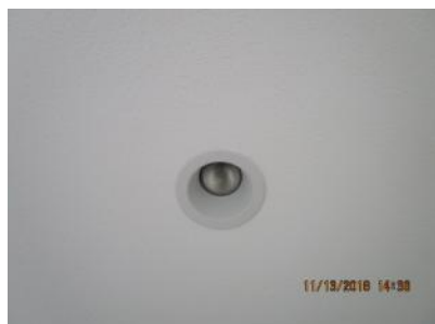
4.39 Recess fixtures appeared generally sound.
