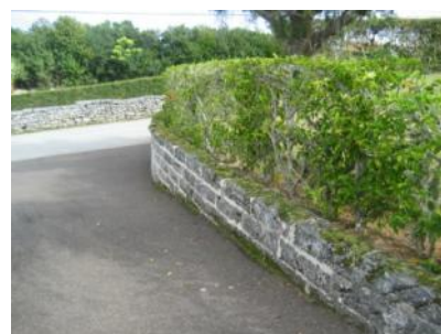
Some vertical cracking was observed in the stone wall but the wall was plumb with no indications of significant movement.
