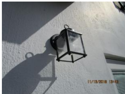
4.90 EXTERIOR Outlets, Fixtures, and Switches
