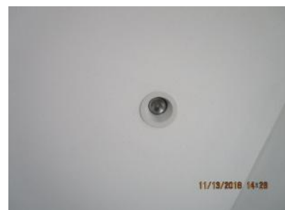
4.17 Recess fixtures appeared generally sound.
