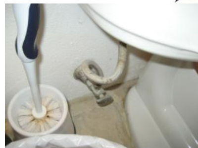
Shut off for master bath toilet was present.
