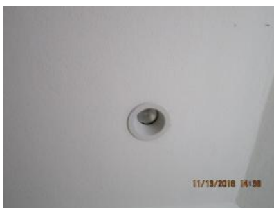
4.46 Recess fixtures appeared generally sound.
