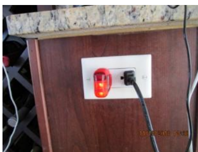
4.25 Counter GFCI receptacle outlet (W) tested ok; appeared generally sound.
