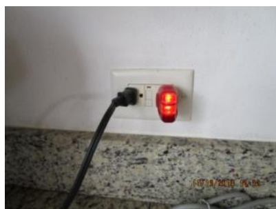
4.30 Counter GFCI receptacle outlet (S) tested ok; appeared generally sound.
