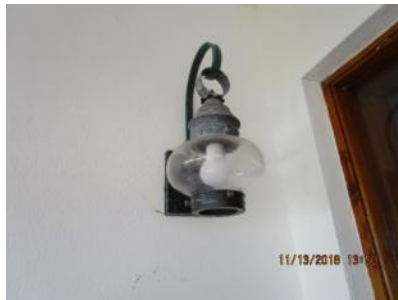
4.96 Main entry fixtures appeared generally sound.
