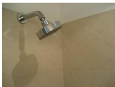
Shower flow and drain tested satisfactorily.
