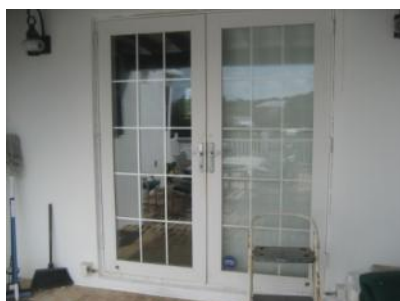
French doors were in satisfactory condition.
