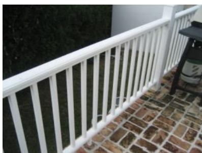
Railing was in satisfactory condition.
