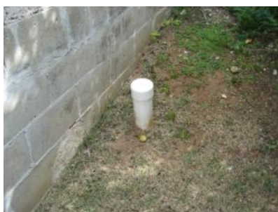
There appeared to be a clean out on the south side of the property.
