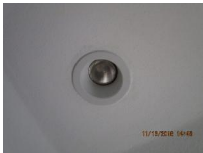
4.72 Recess fixtures appeared generally sound.
