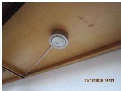
4.33 Under cabinet fixtures appeared generally sound.
