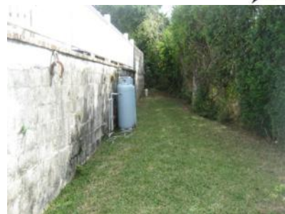
South side of the property was in satisfactory condition.
