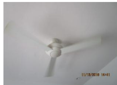
4.56 Ceiling fan appeared generally sound.
