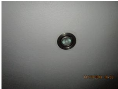
4.88 Recess fixtures appeared generally sound.
