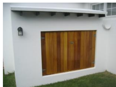
East storage shed was in satisfactory condition.
