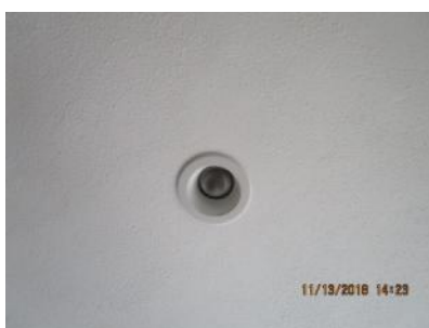
4.4 Recess fixtures appeared generally sound.
