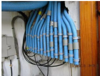
1.4 The Cable/ Data wiring appeared generally sound.
