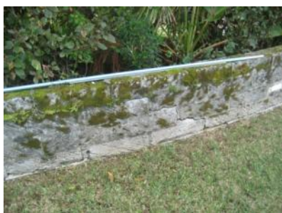
East boundary wall was in satisfactory condition.
