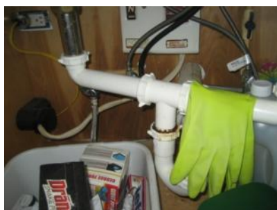
Drain and shut offs for sink appeared to be in satisfactory condition.
