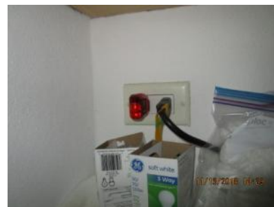
4.20 Counter receptacle outlet appeared generally sound.
