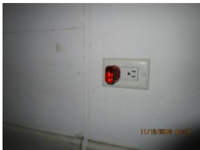
4.43 Closet receptacle outlet appeared generally sound.
