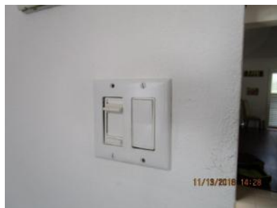
4.18 Switches appeared generally sound.
