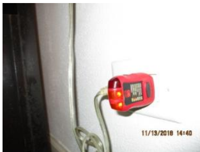
4.52 Receptacle outlet (S) appeared generally sound.
