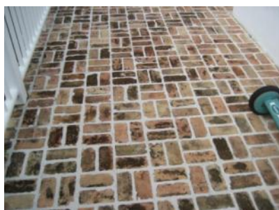
South patio was generally in satisfactory condition.
