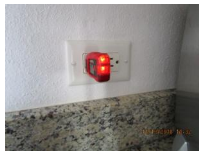
4.29 Counter GFCI receptacle outlet (S) tested ok; appeared generally sound.
