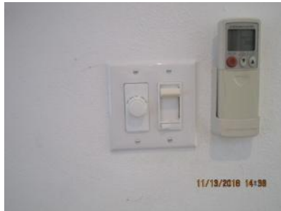
4.48 Switches appeared generally sound.
