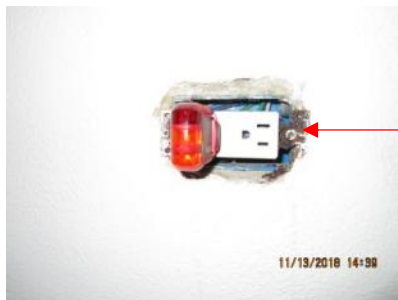
4.51 Receptacle device (W) requires replacement as the device strap has rusted away.
