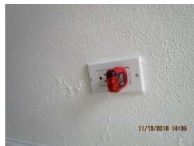
4.38 Receptacle outlets appeared generally sound.
