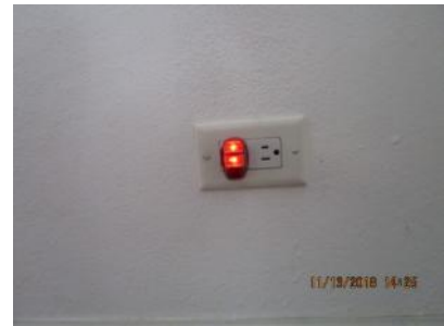
4.8 Receptacle outlet (W) appeared generally sound.
