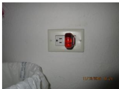
4.21 Receptacle outlet (S) appeared generally sound.
