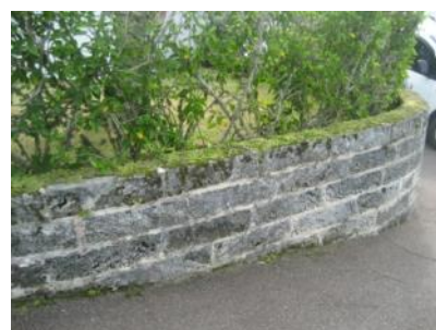
Some vertical cracking was observed in the stone wall but the wall was plumb with no indications of significant movement.
