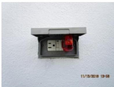
4.94 GFCI receptacle outlet (E) tested ok; appeared generally sound.
