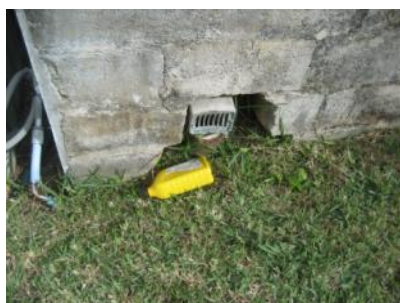
An old cess pit vent was visible at the bottom of the south patio wall.
