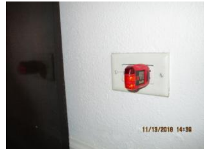
4.50 Receptacle outlet (E) appeared generally sound.
