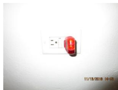
4.86 GFCI receptacle outlet tested ok; appeared generally sound.
