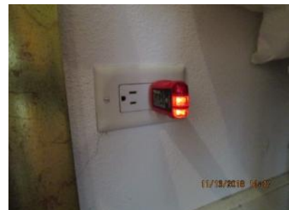
4.71 Receptacle outlet (E) appeared generally sound.
