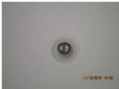
4.9 Recess fixtures appeared generally sound.
