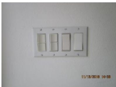
4.40 Switches appeared generally sound.
