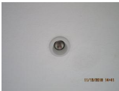
4.55 Recess fixtures appeared generally sound.
