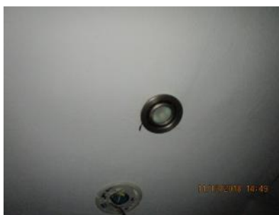
4.76 Recess fixtures appeared generally sound.
