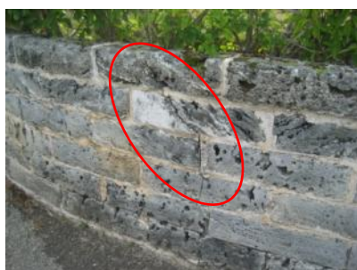
A section of wall near the northeast corner of the property did not appear to be plumb.
