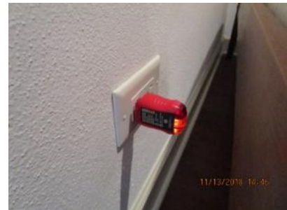
4.68 Receptacle outlet (W) appeared generally sound.
