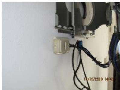
4.54 Receptacle outlet (E) appeared generally sound.
