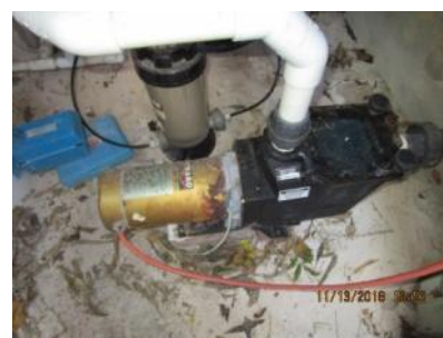
7.18 The filter pump is grounded and bonded as per code.
