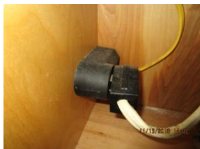
5.11 The receptacle, cord and cap appeared generally sound.
