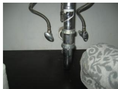
Shut offs and drain for the lower bathroom sink appeared to be in satisfactory condition.
