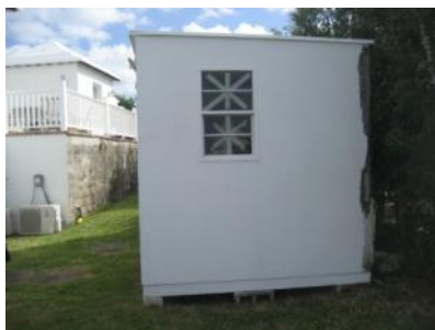
Shed on the south side of the property.
