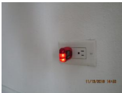
4.79 Receptacle outlet (S) appeared generally sound.
