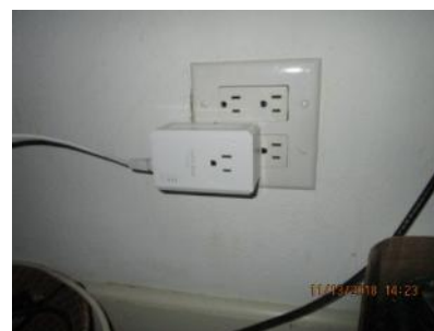
4.2 Receptacle outlets west (W) appeared generally sound.
