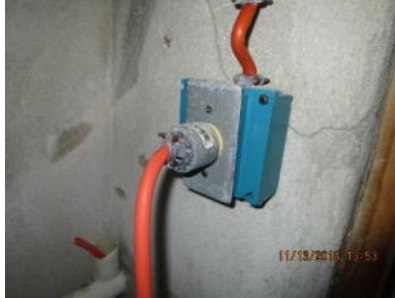
7.20 Receptacle outlet appeared generally sound.
