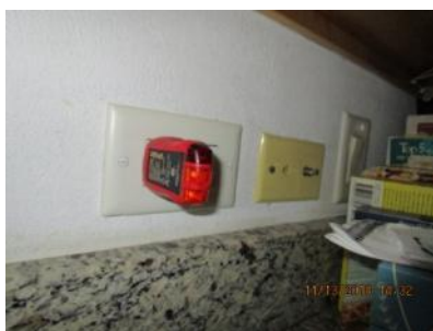
4.31 Counter GFCI receptacle outlet (S) tested ok; appeared generally sound.
