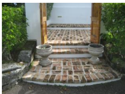
Entrance steps and landing were in satisfactory condition.
