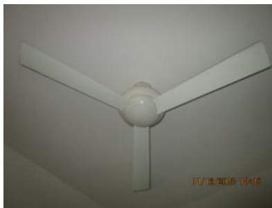
4.73 Ceiling fan appeared generally sound.
