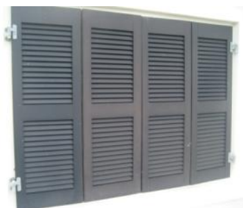
The shutters generally appeared to be in satisfactory condition.
