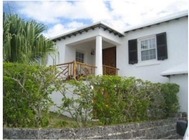
View from driveway
