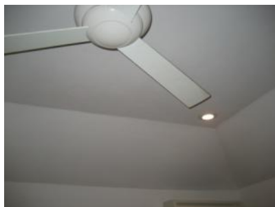
The ceiling was in satisfactory condition.
