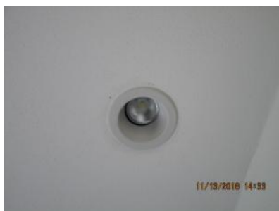
4.34 Recess fixtures appeared generally sound.
