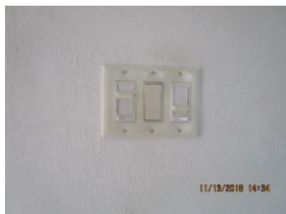
4.36 Switches appeared generally sound.
