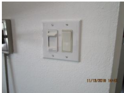
4.57 Switches appeared generally sound.
