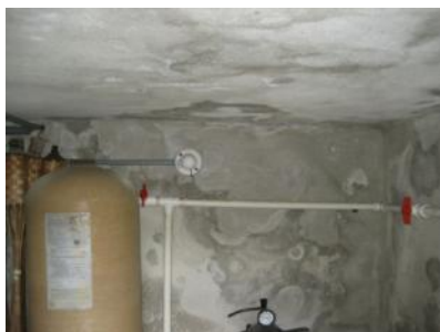
Ceiling appeared to be in satisfactory condition.
