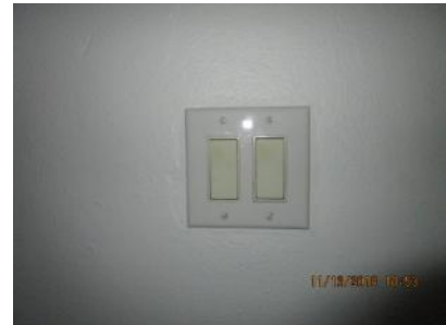
4.89 Switches appeared generally sound.
