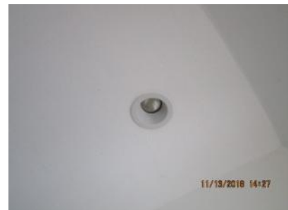
4.11 Recess fixtures appeared generally sound.
