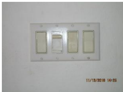
4.12 Switches appeared generally sound.
