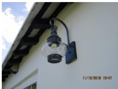
4.93 Wall Fixture (E) appeared generally sound.
