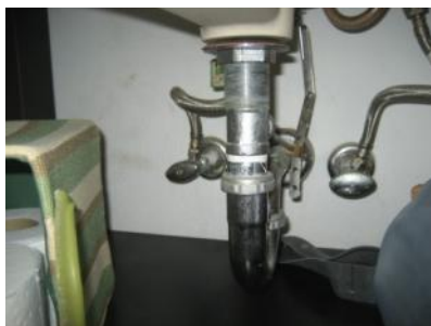
Shut off and drains for the hallway bathroom appeared to be in satisfactory condition.
