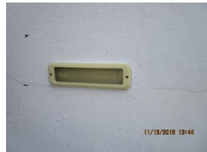
4.92 Recessed fixtures (N) appeared generally sound.
