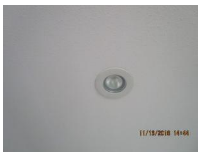
4.64 Recess fixtures appeared generally sound.
