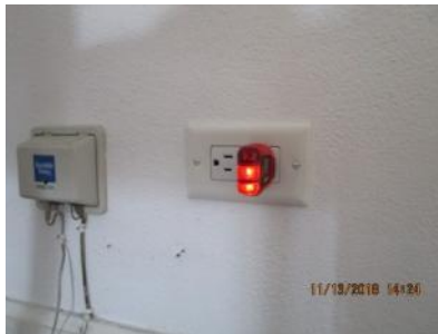
4.7 Receptacle outlet (E) appeared generally sound.
