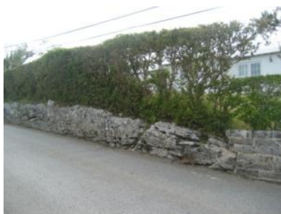
North boundary wall.
