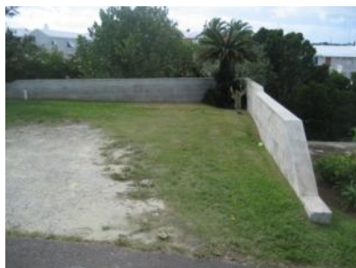
West yard was in satisfactory condition.
