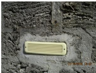
4.100 Recessed louvered fixtures (S) appeared generally sound.
