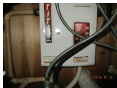
5.10 A tankless water heater located under the kitchen sink appeared generally sound.
