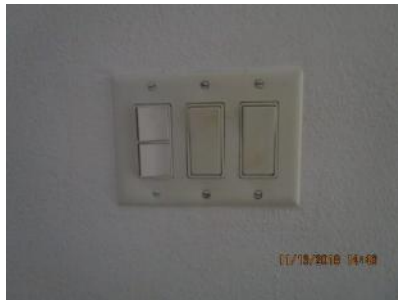
4.66 Switches appeared generally sound.
