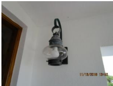
4.97 Main entry fixtures appeared generally sound.
