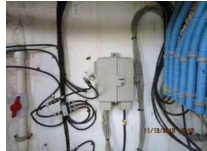
1.3 The incoming BTC terminal box appeared generally sound.
