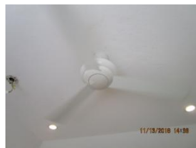
4.47 Ceiling fan appeared generally sound.
