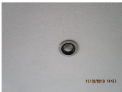
4.82 Recess fixtures appeared generally sound.
