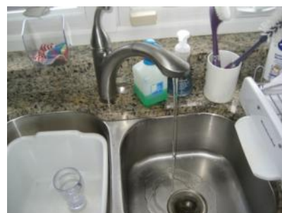
The kitchen sink flow and drain tested satisfactorily.
