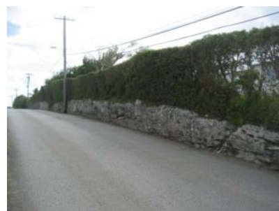
North boundary wall was generally in reasonable condition.
