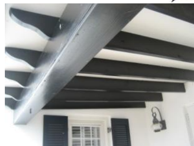
Framing over porch was in satisfactory condition.
