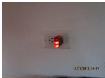
4.42 Receptacle outlet (N) appeared generally sound.
