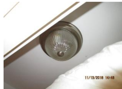
4.74 Closet fixture appeared generally sound.
