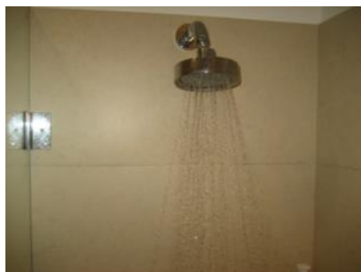
Shower flow and drain tested satisfactorily.
