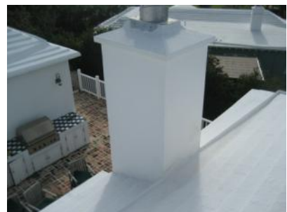
Chimney was in satisfactory condition.
