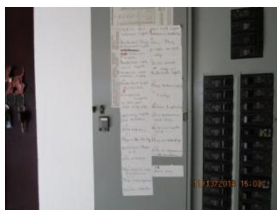
3.3 Panel directory was complete; appeared accurate.
