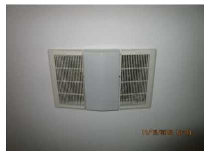
4.65 Heat, Vent, Light tested ok; appeared generally sound.
